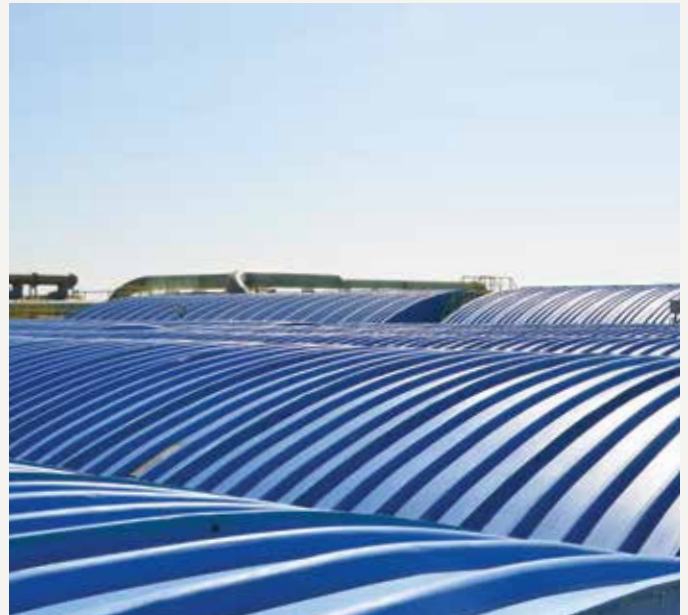
After upgrading in 2015
